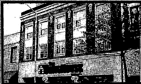
ST. MORITZ APARTMENTS 4513 University Way N.E. • 632-4500
