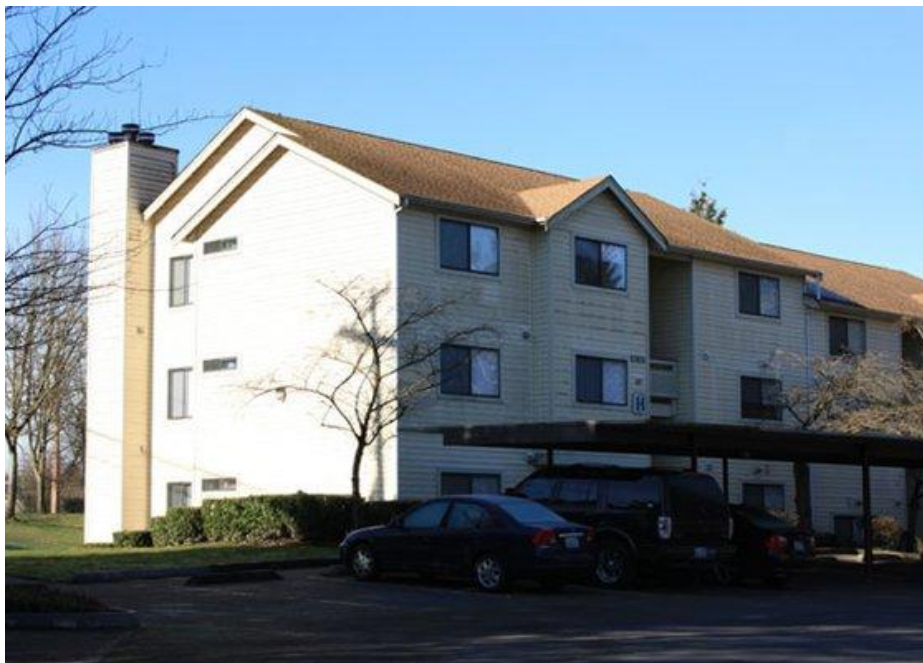
Figure 2. A student residence building at the complex
