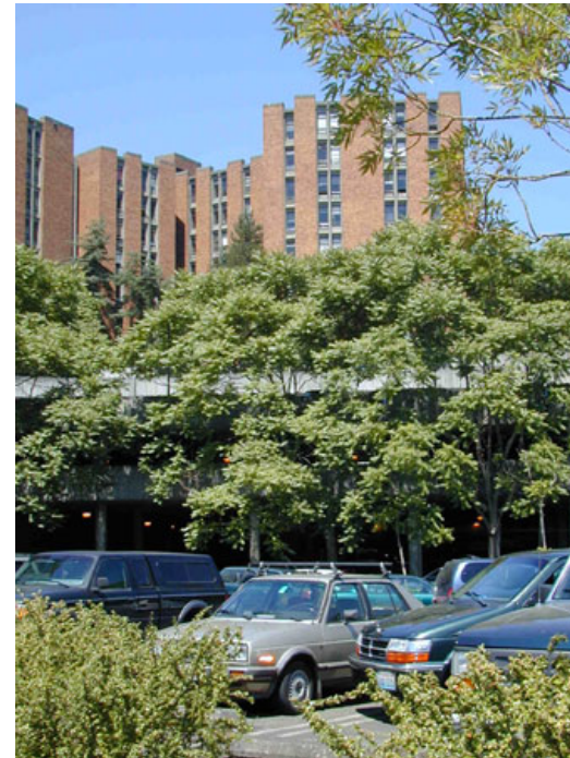
Structured Parking at Padelford
