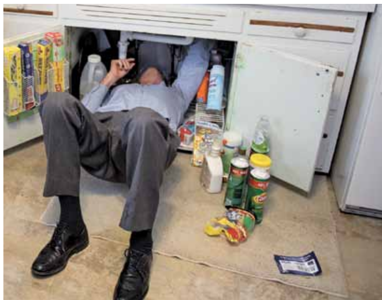
In homes and under sinks like this one in Flint, Edwards, an environmental engineer, looks for clues as to why the tap water in this particular house has high levels of lead.
